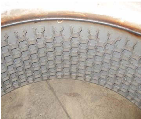
Hexmesh before castable material has been installed.
