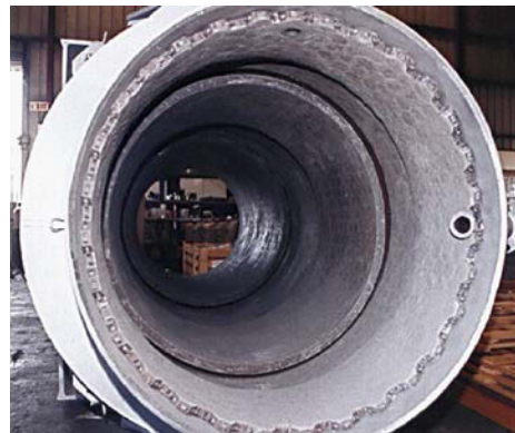
After castable material has been installed.
